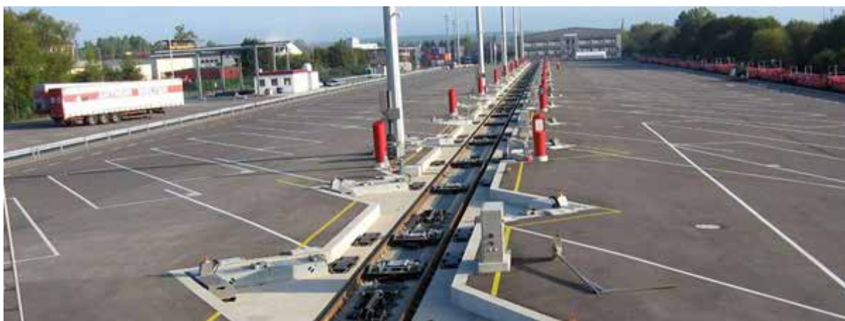
Rys. 3.14 Terminal systemu Modalohr [60]
